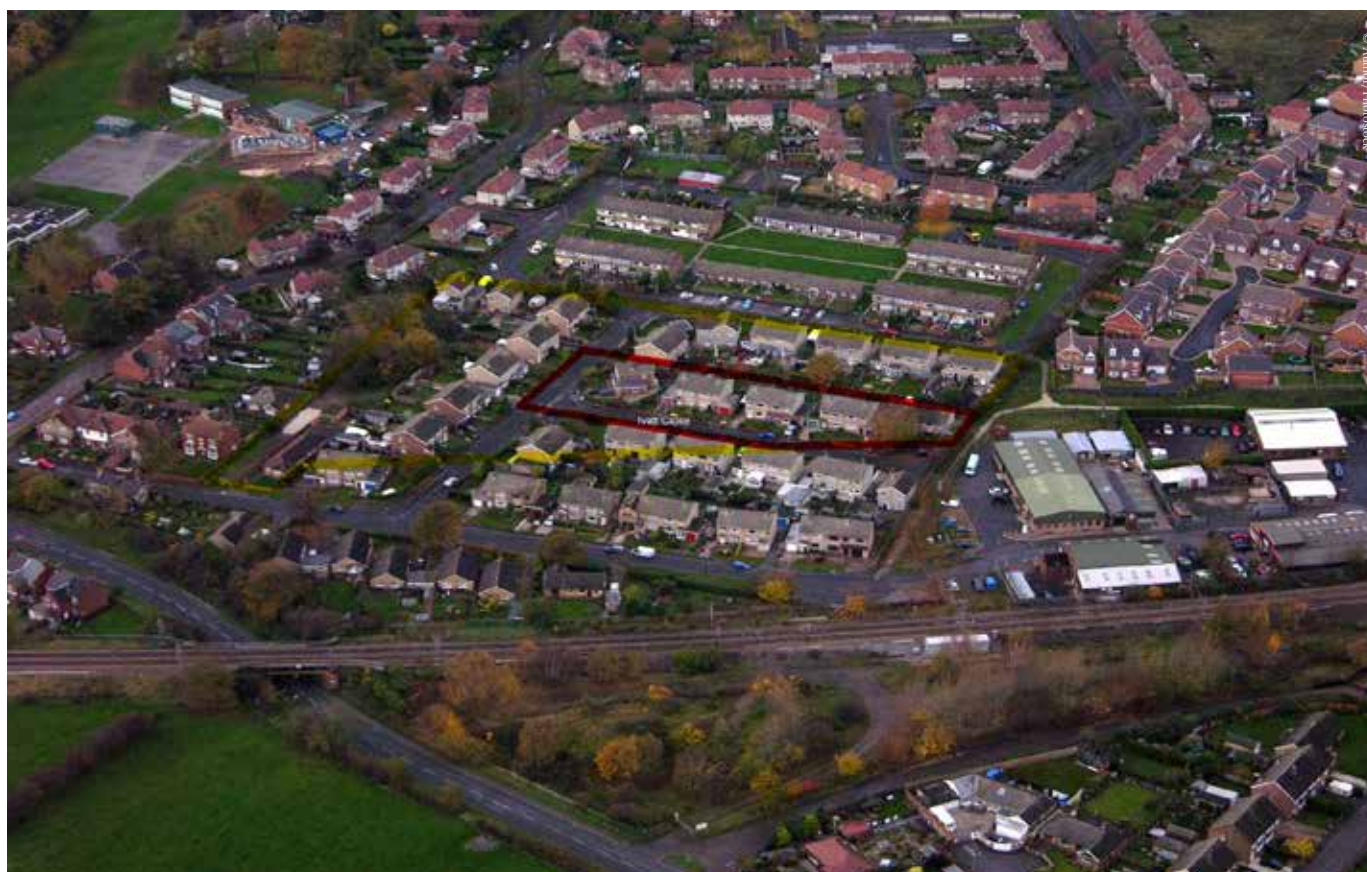
Bawtry Gasworks -developed site – present day
