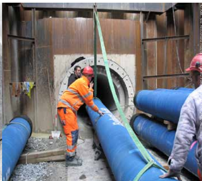
Introduction of the new drinking-water pipe into the diverted channel
