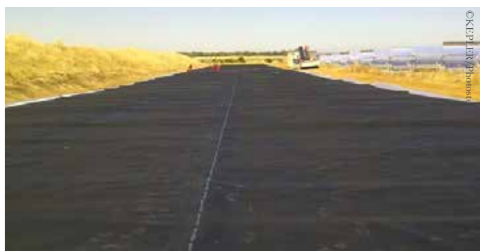
Positioning of the 1.5mm high density polyethylene sheet
