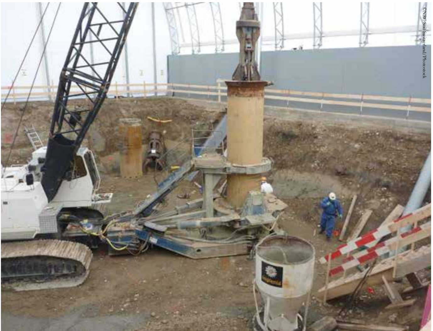
Pollution excavation under the protective cover by means of large diameter drilling.
