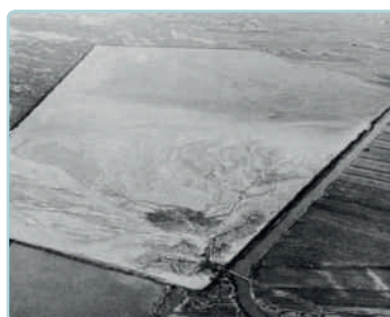
The construction of the industrial port: sediment tanks for the realization of the third industrial area
